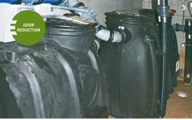
According to EN1825-1, grease traps must be installed if there is a risk that more than insignificant amounts of grease are flushed out into the drain. Ozone eliminates odors and microorganisms very quickly and efficiently without leaving behind any chemical byproducts.
